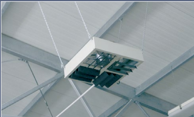
installation of a ceiling-mounted fan
