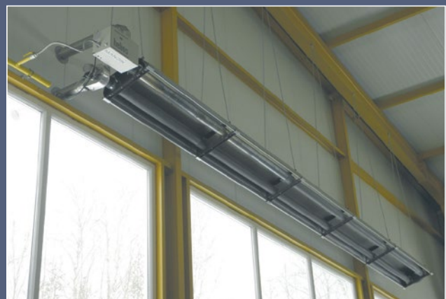
installation of the Helios infrared heater
